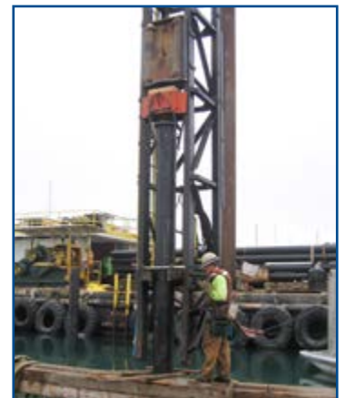
Installation of Piles
