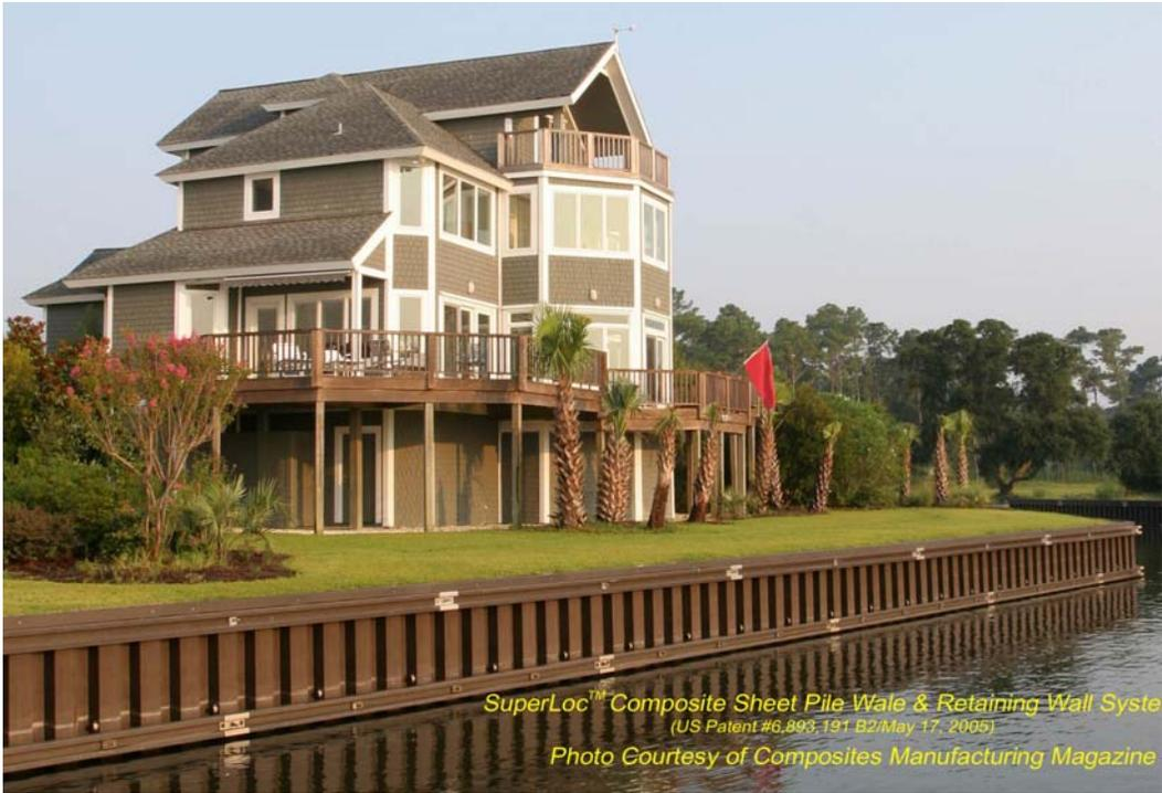
**Figure 7.0 Superloc™ Sheetpile system with the polyurethane cap**
