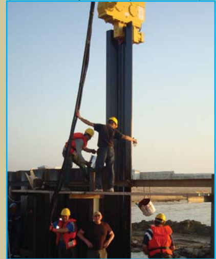
Example of Driving SuperLoc™ Sheet Piles
