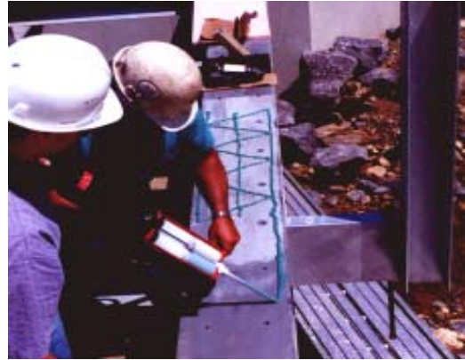
High performance adhesive bonding is applied to beam surface.
