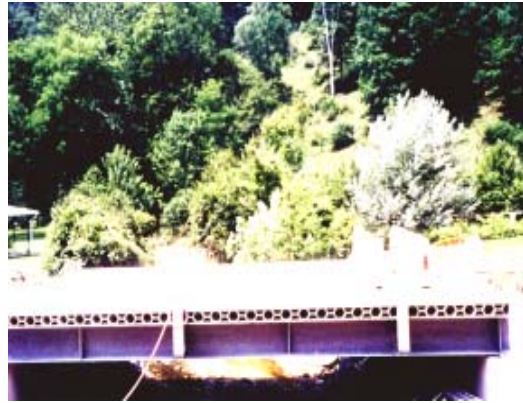
On-site assembly takes only a few hours for completion.
