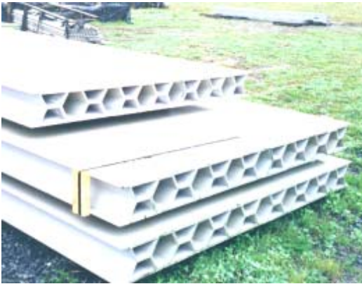
Deck panels arrive at site, ready for installation.
