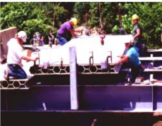
Prefabricated Superdeck™ is installed using minimal equipment.
