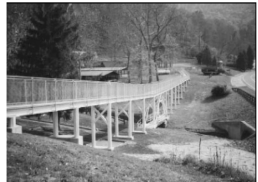
Pultruded Component Handicap Ramp Beacon Lodge
